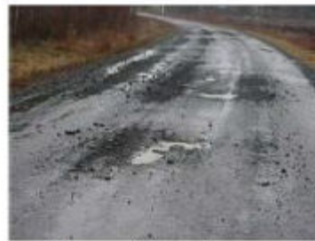
Freeze-thaw damage
